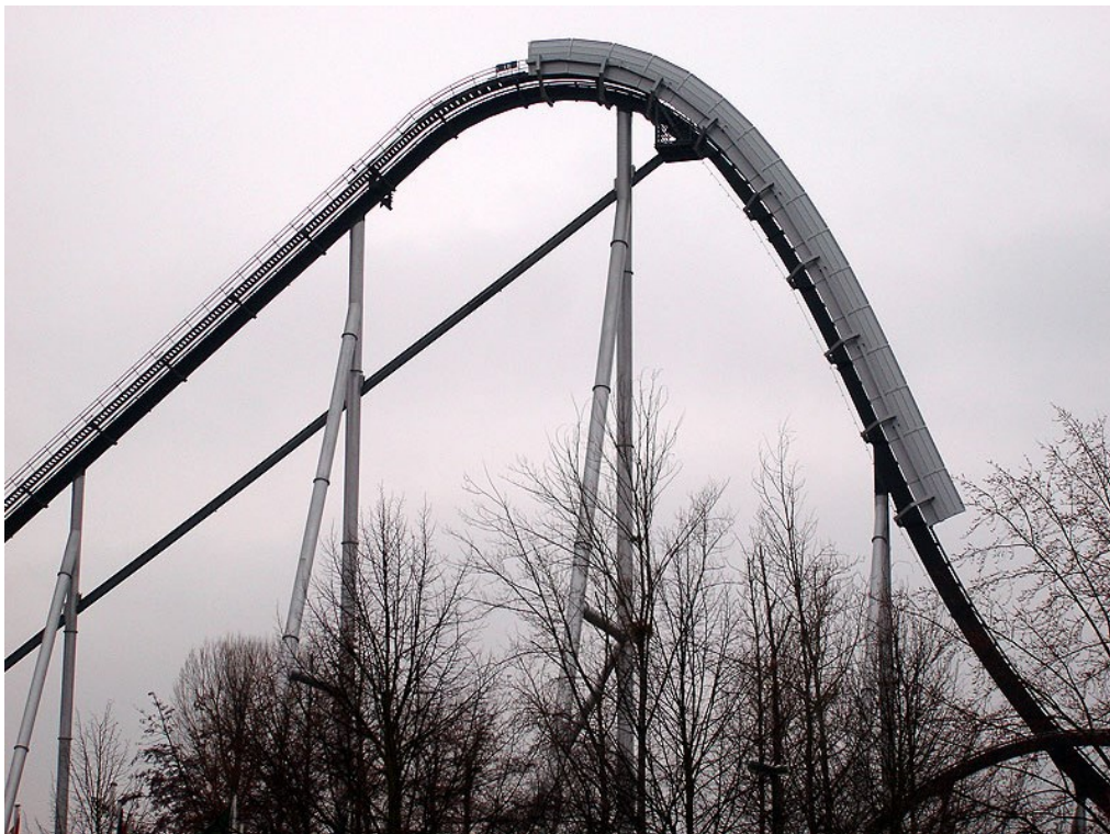
Figure 38: Noise protection wall added several years after opening [Fig. 25] (Silver Star – Europa Park)
