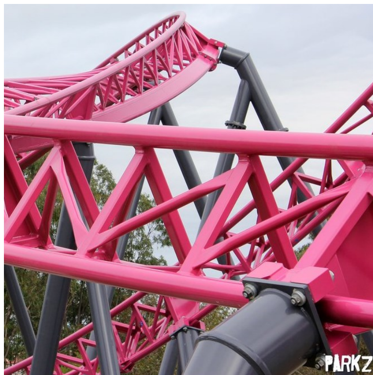
Figure 26: MACK flattened diagonal ends and thicker spine (background) [Fig. 17] (DC Rivals HyperCoaster – Warner Bros. Movie World)
