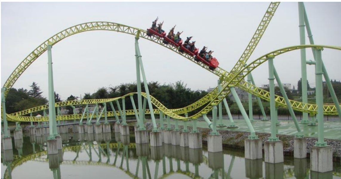
Figure 29: Spined track and spineless track on the same coaster [Fig. 18] (Kawasemi – Tobu Zoo)
