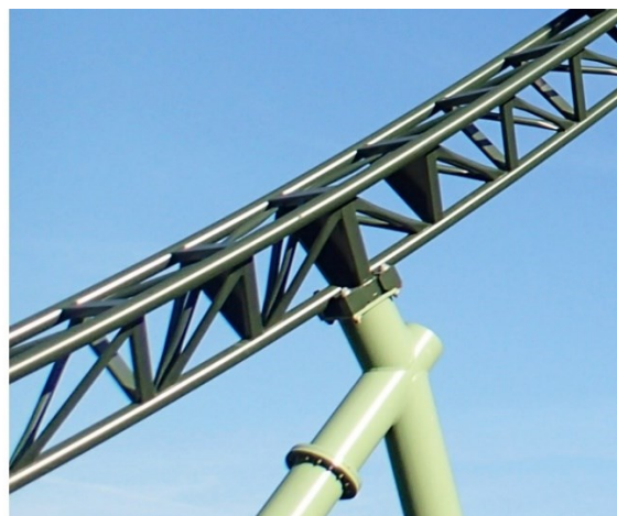
Figure 30: Support connections by Intamin (left) (Expedition GeForce – Holiday Park) and MACK (right) (Helix – Liseberg)
