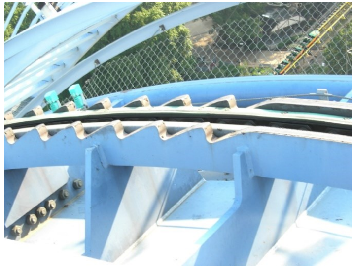
Figure 12: Anti-rollback teeth [Fig. 9] (Griffon – Busch Gardens Williamsburg)
