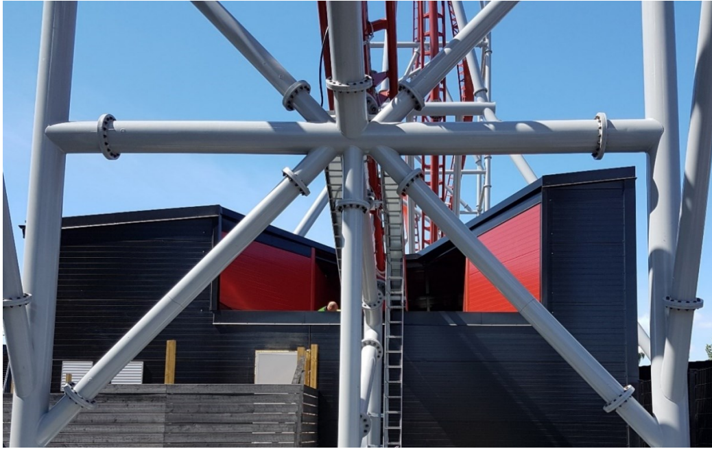
Figure 33: Flanges in supports with bolted connections (Hype – Särkänniemi)
