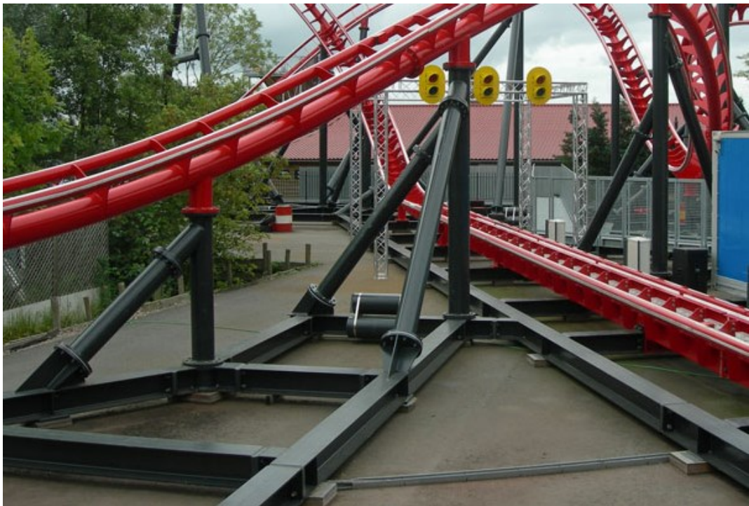
Figure 37: Steel lattice used as foundations [Fig. 24] (Formule X – Drievliet Family Park)
