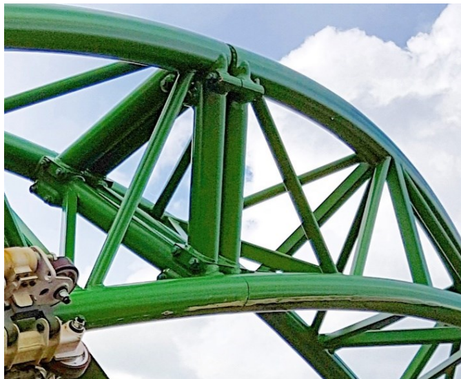
Figure 34: Bolted connection between track pieces (Junker – Power Park)
