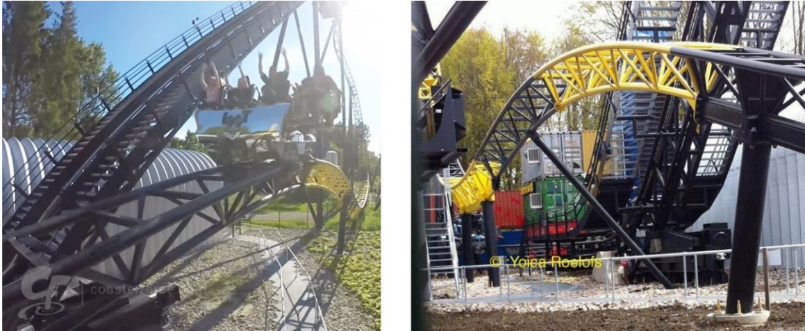
Figure 32: Airtime hill without (left) [Fig. 20] and with added lateral support (right) [Fig. 21] (Lost Gravity – Walibi Holland)
