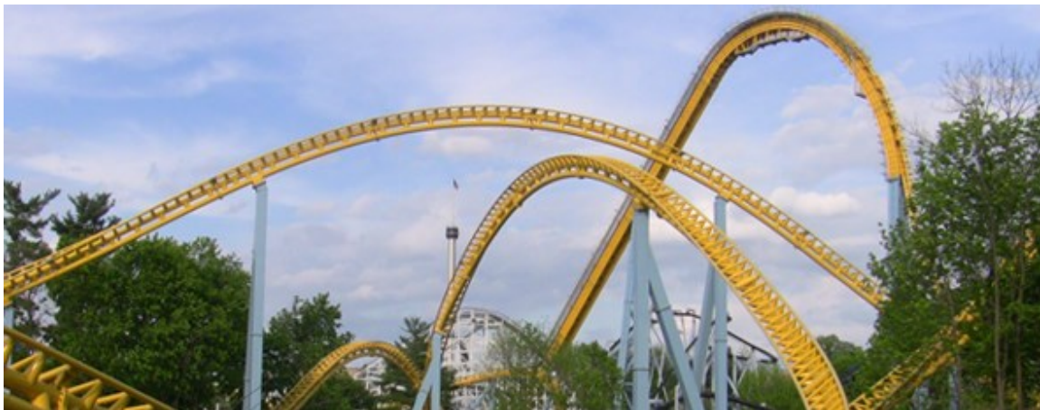
Figure 31: Rigid spine and concave shape allow long spans [Fig. 19] (Skyrush – Hersheypark)
