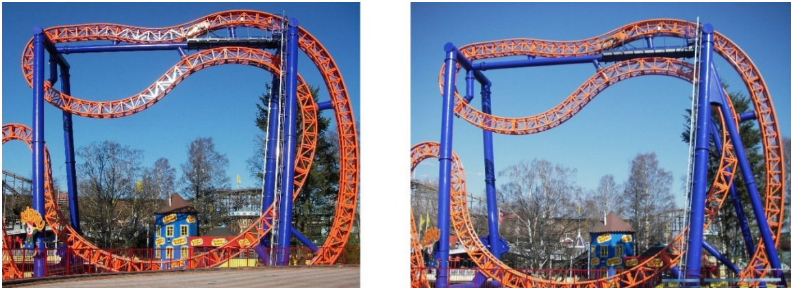
Figure 23: Kirnu in 2007 (left) and with added supports in 2008 (right)
