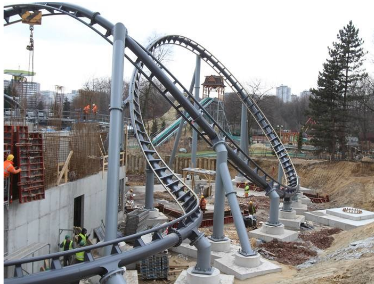
Figure 15: Example of track simultaneously rotating around all axes [Fig. 12] (Lech Coaster – Legendia)
