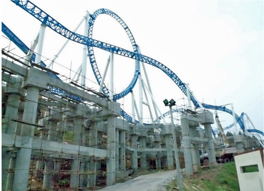
Figure 36: Custom concrete footers used in a copied layout [Fig. 23] (Crazy Coaster – Loca Joy Holiday Theme Park)
